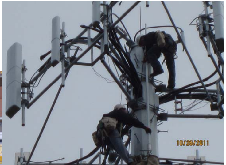
OUR ANTENNAS FINALLY BEING INSTALLED!
