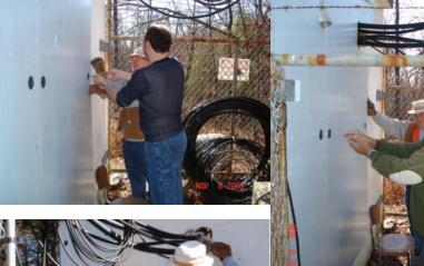
Above: Jim, KC2OGK, fastens insulating panels to the walls of the repeater shack.
