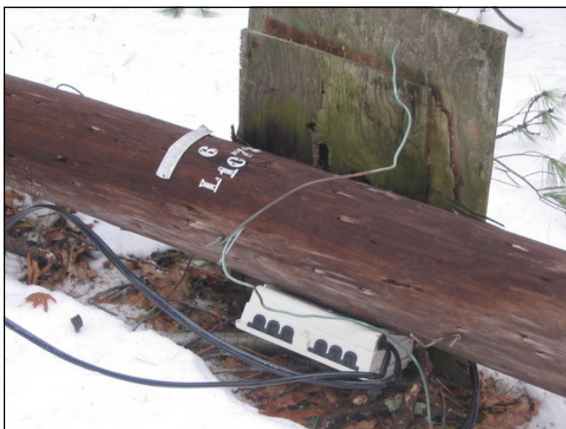
Downed pole with telephone box.
