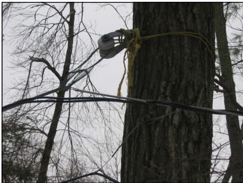
Damage to the AC Line.
