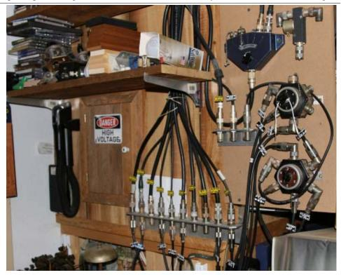
The Ham Shack of Stan, WA2UET, has well organized antenna leads and grounding for static and lightening discharge. WA2UET Photo
